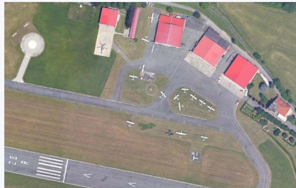
Apron, hangar e area atterraggio HEMS — vista aerea / HEMS landing area — aerial view
